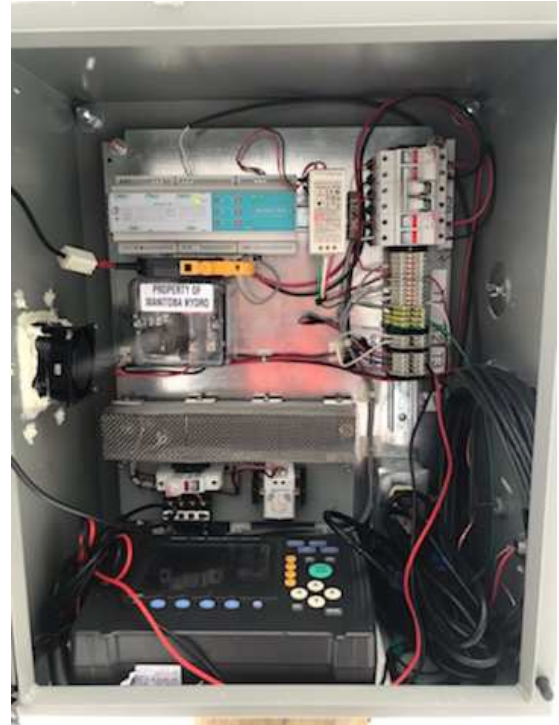
Pictures – 8 and 9 HIOKI metering cabinet on the same pole with MVROT
