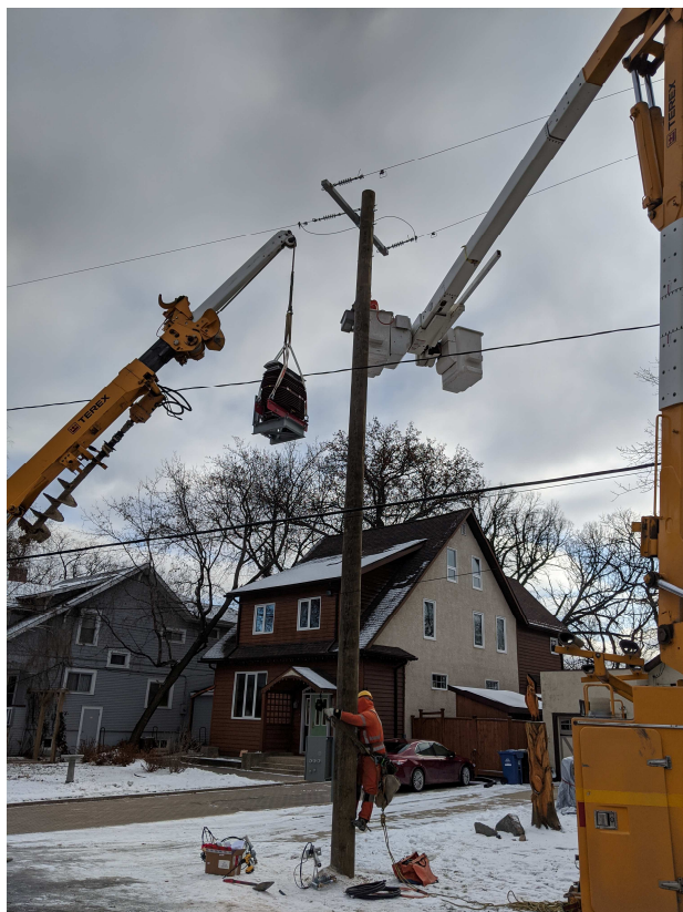
Picture-5 lifting MVROT on 50’ tall pole
