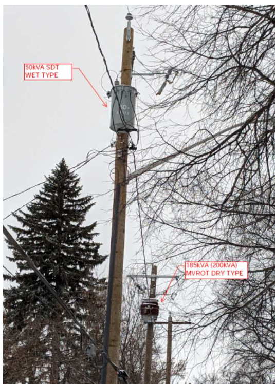
Pictures-10 and 11 view showing 4 times larger power capacity of 185kVA MVROT versus Oil filled 50kVA SDT, physical sizes are almost the same
